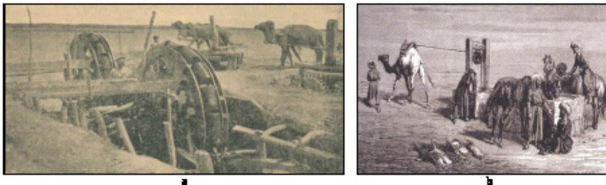
Picture 5 – a) Camel-driven water wheel. Left bank of Syrdaria, end of XIX c. Photography by M.Diakov (Aleksandrov, 1920: 19); b) the camel-driven water lift from a well.
