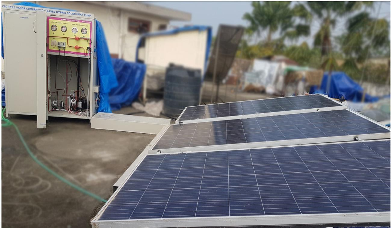
Figure 2 – Photographic view of the heat pump-based PV-T water heater system installed at the SEC
