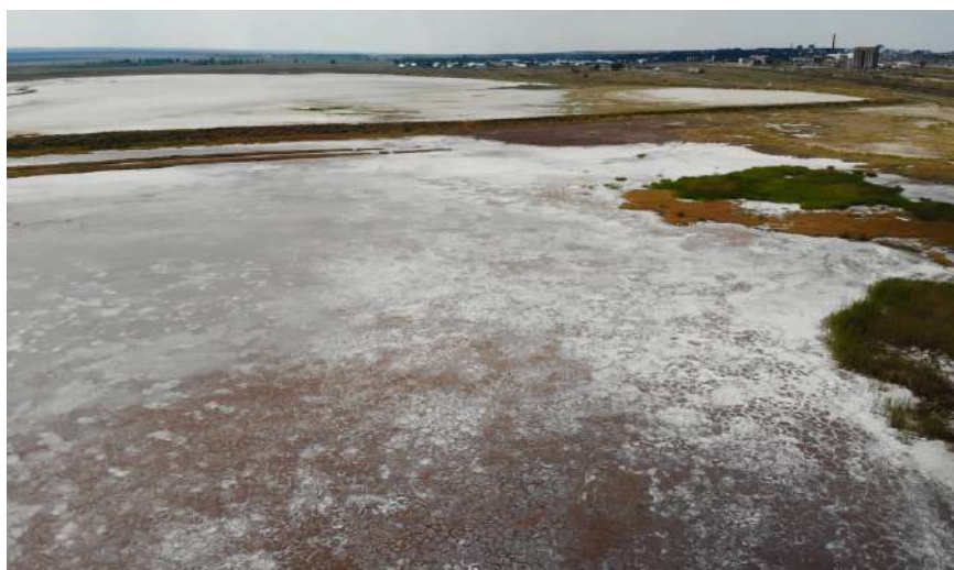
Figure 1 – Present condition of the "old" sludge collectors from the boric acid production of the Alga Chemical Factory
