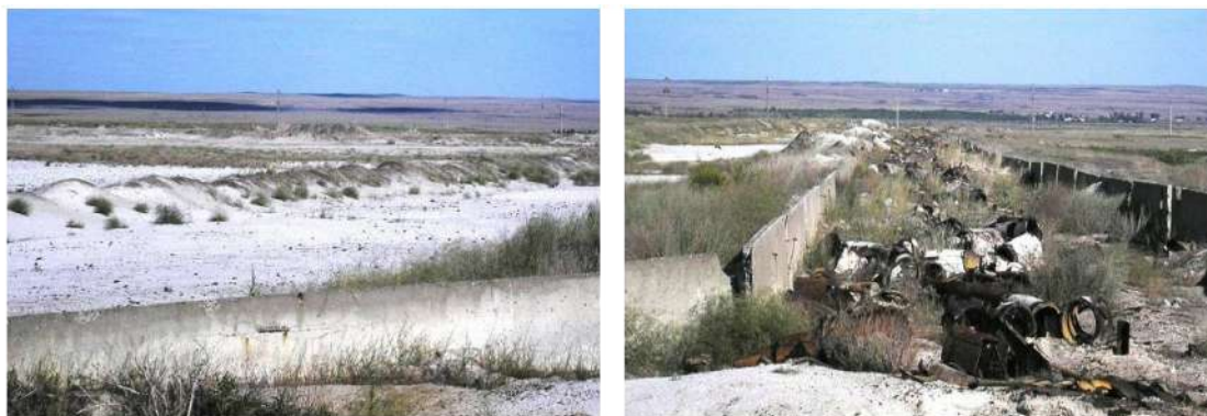
Figure 4 – Pipeline condition with traces of emergency discharges
